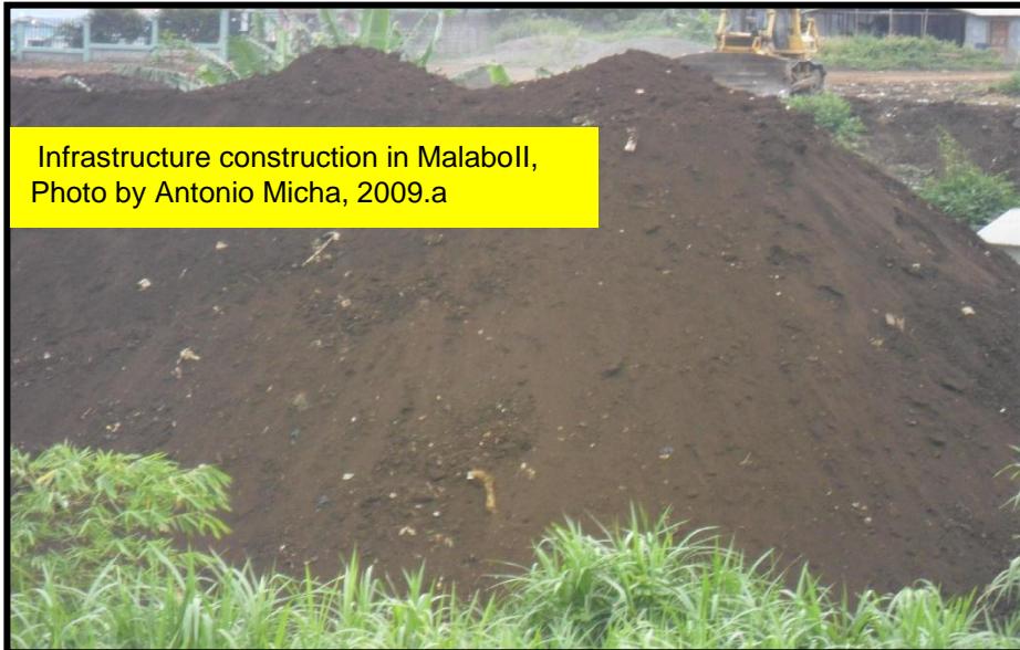
Infrastructure construction in Malaboll, Photo by Antonio Micha, 2009.a
